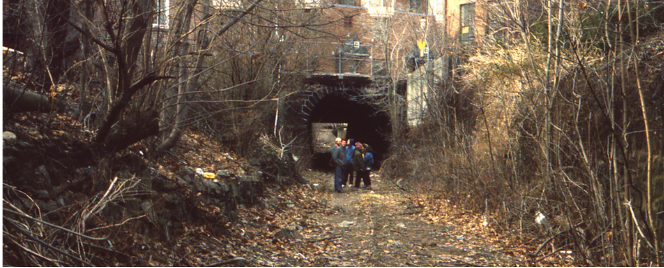
Current condition of adjacent Canal Trail
